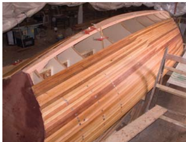
Strips are held in place temporarily by screws and penny washers.
